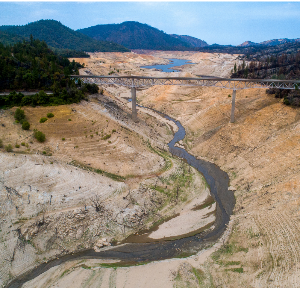
Top: Lake Oroville at the Enterprise Bridge in July 2021
