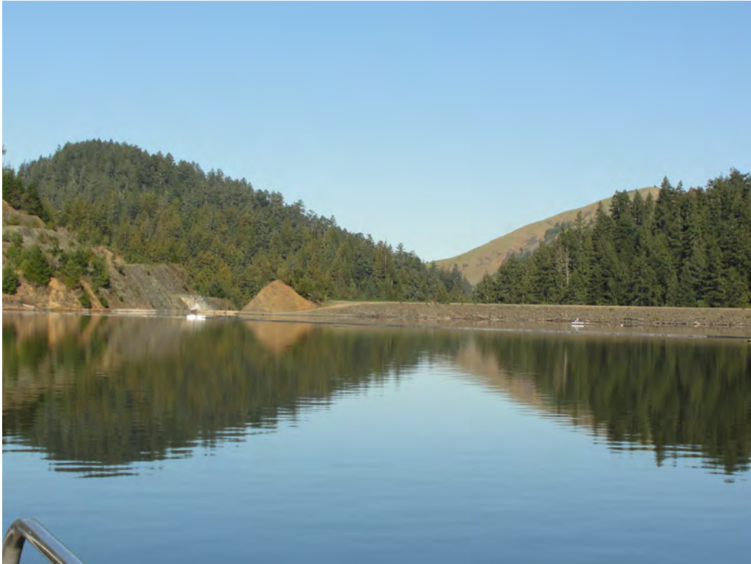
Peters Dam (Kent Lake), facing downstream, 2015.
