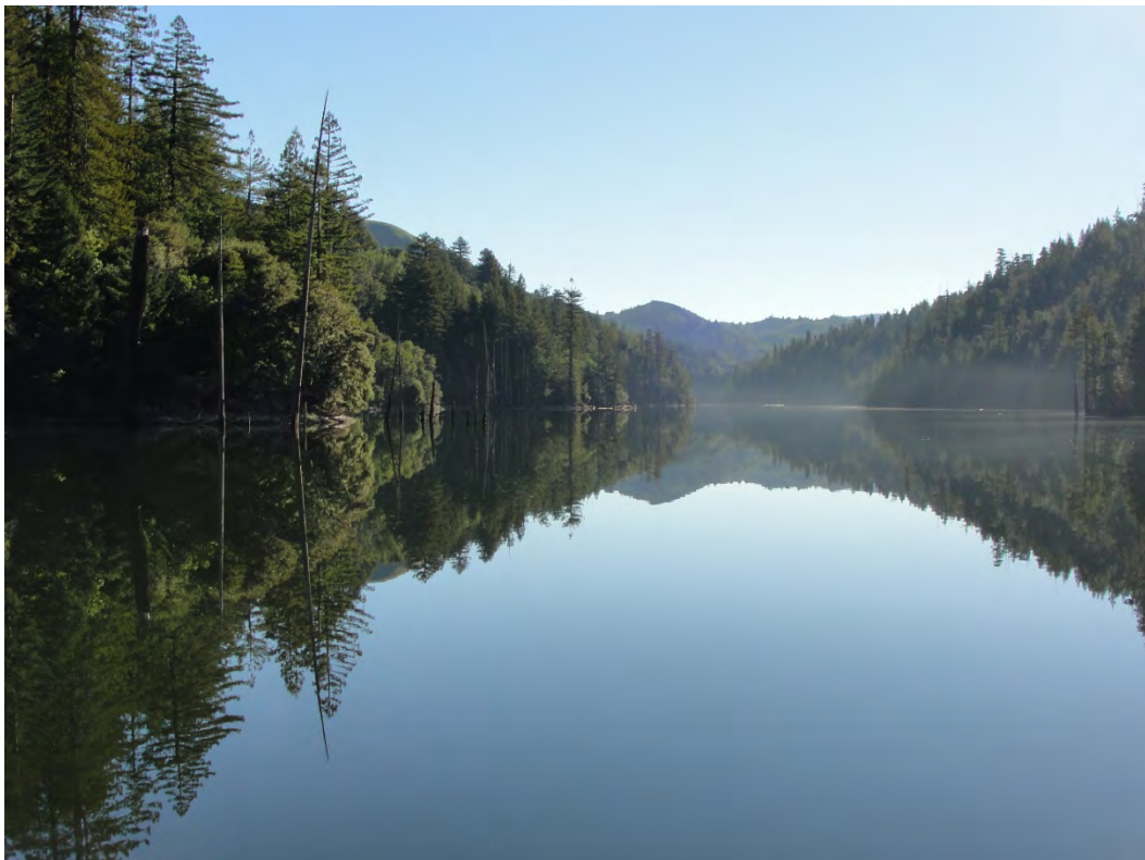
Peters Dam (Kent Lake), facing upstream, 2015.
