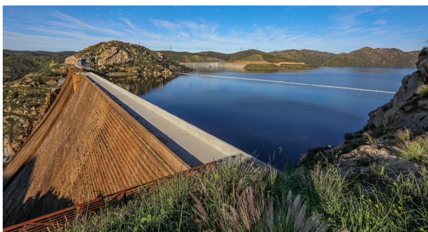
The City of San Diego's San Vicente Dam, constructed in the 1940s, was raised 117 feet as part of San Diego County Water Authority's (SDCWA's) emergency storage project, more than doubling the reservoir's capacity and improving the drought resiliency of a region having relatively little local surface water or groundwater storage capacity. The enlargement was completed in 2014. Photo credit: SDCWA
