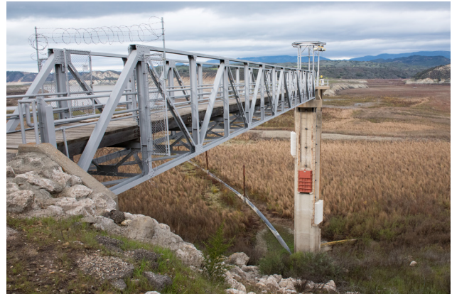
A dry Lake Cachuma in February 2017. The temporary pipeline seen here entering the inlet tower to the Tecolote Tunnel connected a barge-mounted emergency pumping plant on the lake to the inlet. The dry lakebed illustrates lingering Central Coast drought impacts that were not mitigated by a wet Water Year 2017. It was not until early 2019 that lake levels recovered sufficiently to permit decommissioning of the temporary facilities.
