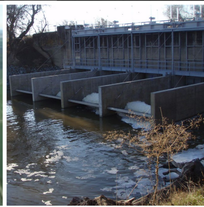
Knights Landing Outfall Gates
