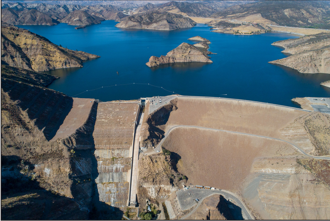
An aerial view of the gated and emergency spillways at Pyramid Dam and Lake, a reservoir near Castaic in Los Angeles County. Source: Department of Water Resources
