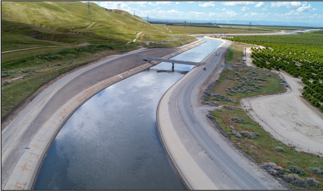
A section of the California Aqueduct that conveys water between the Buena Vista and John R. Teerink Pumping Plants within Kern County. Source: Department of Water Resources
